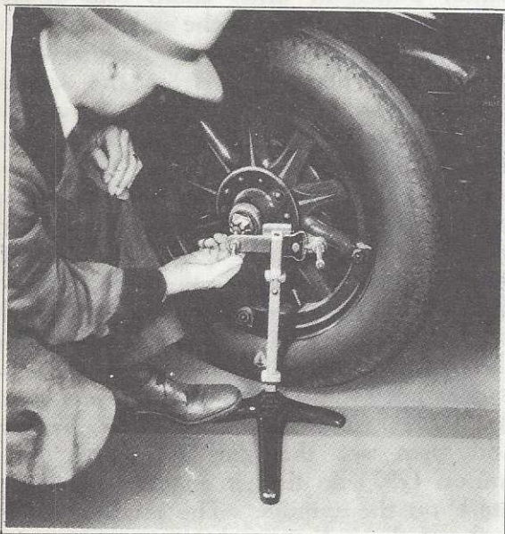
Illustration 1-17—Checking Caster of Front Wheels with Bear Axle Gauge (1st position)
