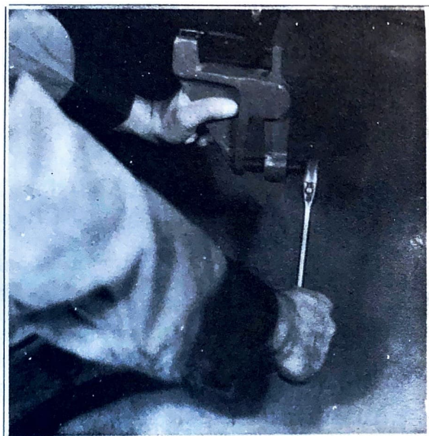
Illustration 10-3—HM-490 Tool for Removing Shackle Bolts in Front End of Front and Rear Springs
